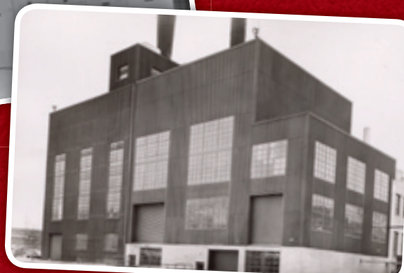
The boilerhouse was added in the 1950s to accommodate the three 400-pound boilers.
