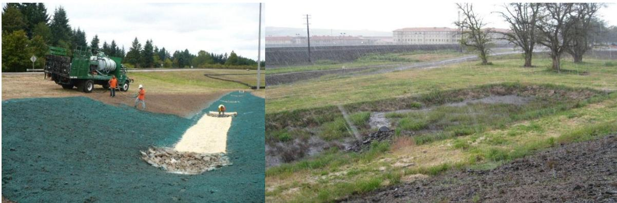
*Two examples of water quality treatment installed by ODOT. On the left, a vegetated water quality swale at the interchange of I-5 and I-205 near Portland. On the right, a water quality pond along I-84.*
