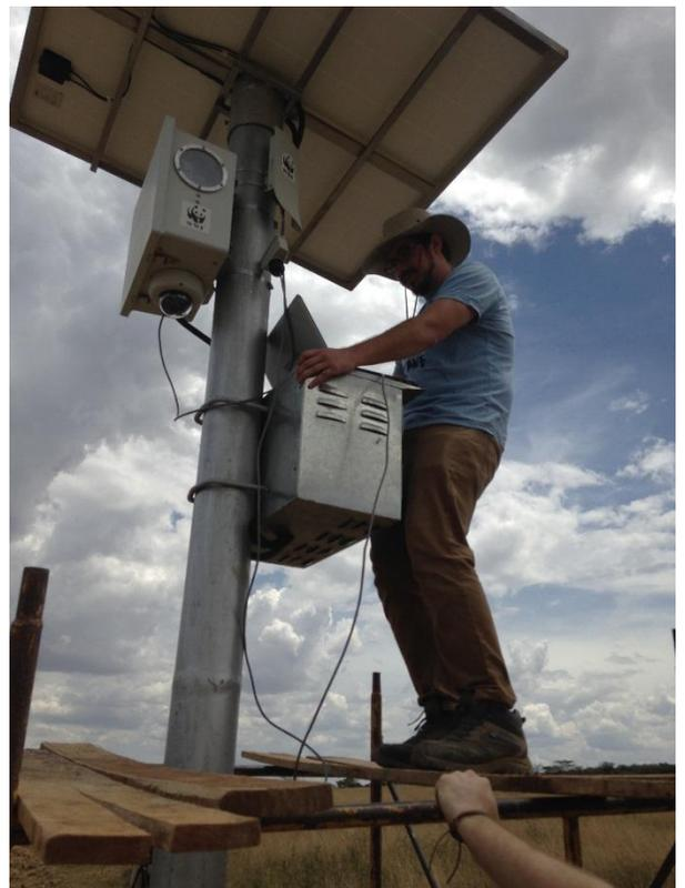
Fig. 1. Installing FLIR cameras with solar panels, Avigilon software, batteries, and radios to send the data to an operations center in Kenya.
