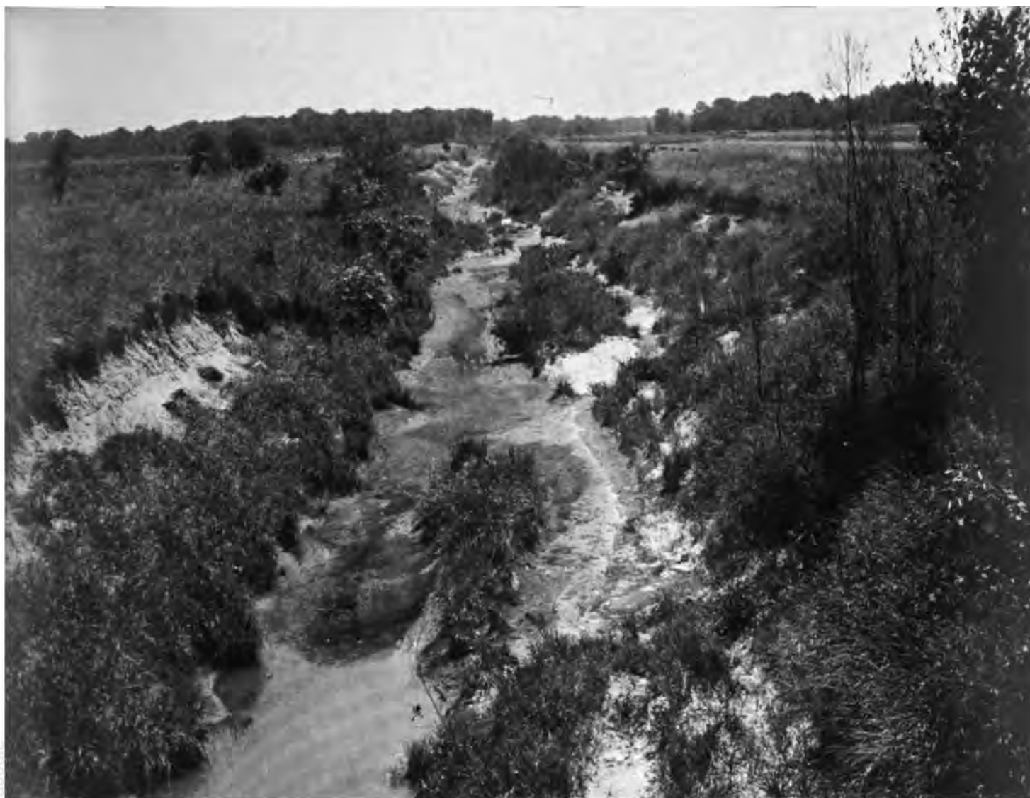
Failure to provide bank protection on this channel leads to excessive erosion
