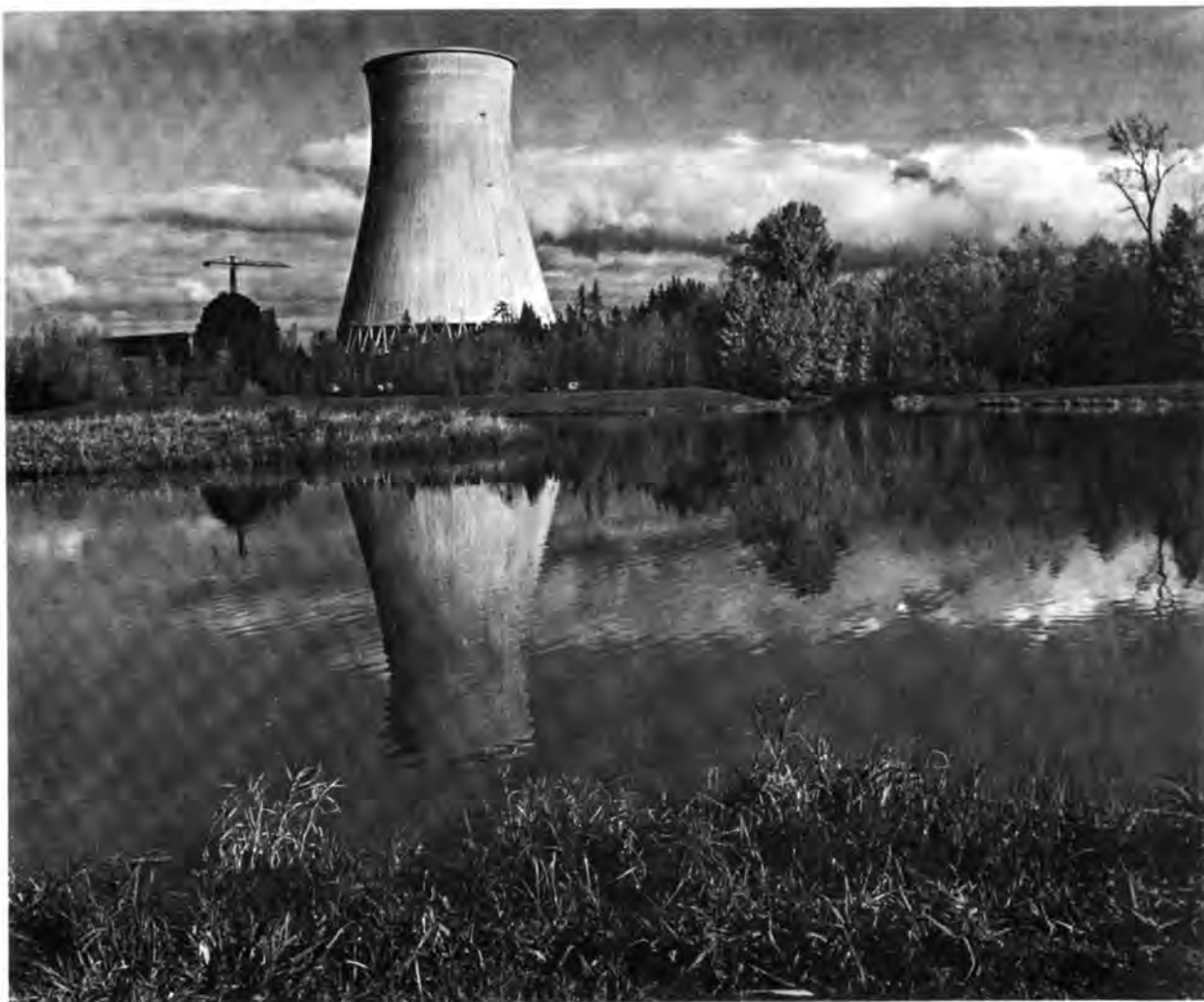
Cooling tower on Trojan Nuclear Plant prevents discharge of heat into the Columbia River
