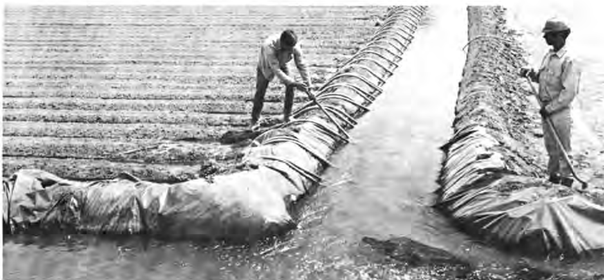
Siphon tubes take water from farm ditch into crop rows in California's Central Valley
