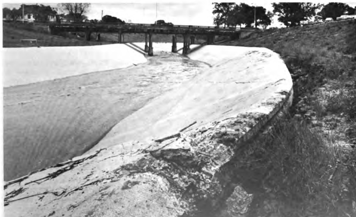
This concrete channel lacks esthetic beauty and requires frequent maintenance
