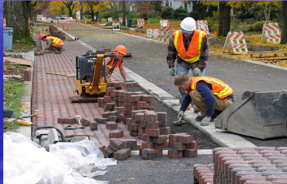
Installation of permeable pavers Courtesy of Portland, BES
