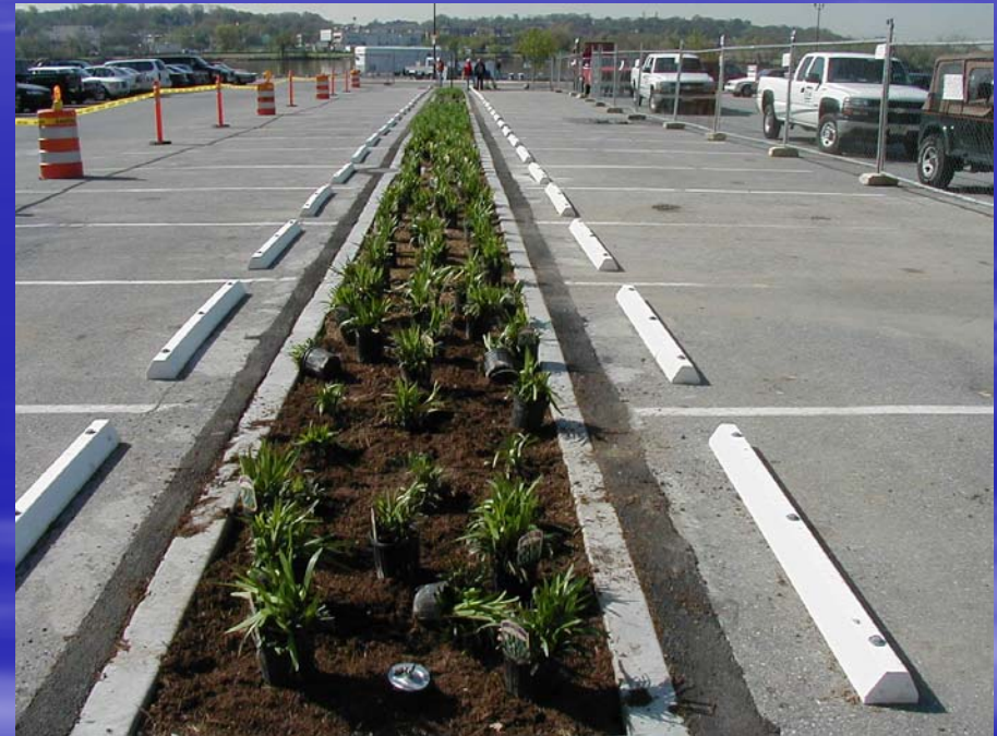
Navy Yard Bioretention. Photo courtesy of LID Center.
